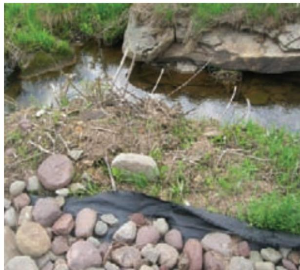
Geotextiles are fabrics used for the stabilization of soil and other material. They keep these materials in place for heavier and longer use. They can also be used in road and bank stabilization. The manufacturer's directions should be followed in their use. Contact a logging or forestry equipment supplier for sources of these materials.
